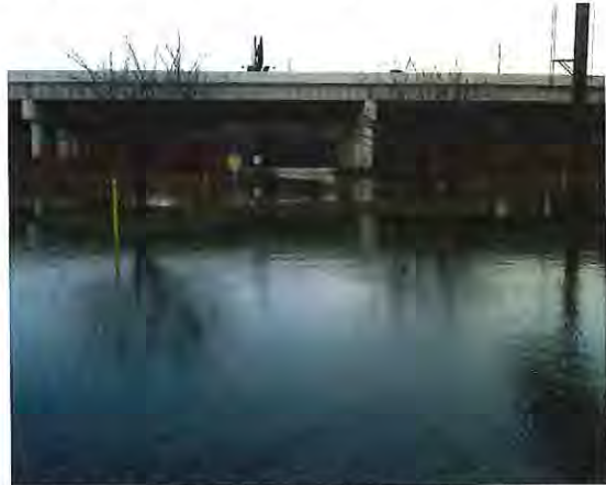
Figure 44. Example of Flooding to the Parking Area at the Wilmington Training Center Flooding
