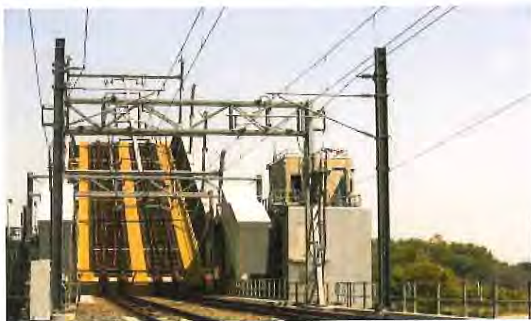
Figure 42. Niantic River Bridge (Amtrak, 2015)
