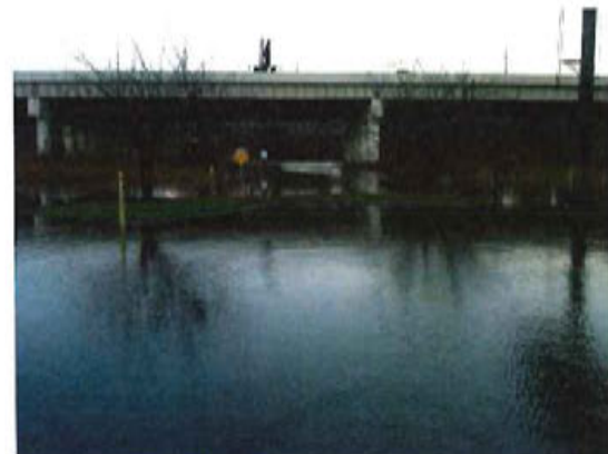
Figure 21. Flood Waters below I-95 Overpass at Access Road Preventing Access to Training Center
