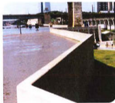
Photo Credit: U.S. Army Corps of Engineers ( mvs.usace.army.mil/Missions/Flood-Risk-Management )
