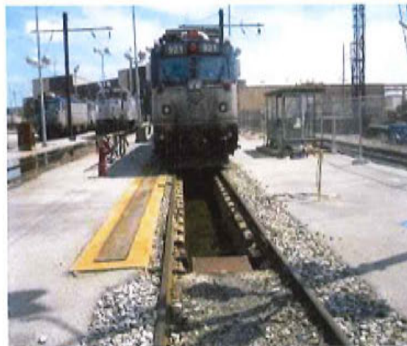
Figure 15. Electric Locomotive above Pit with Standing Water
