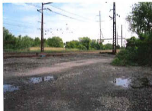
Figure 43. Northern Approach of Track Segment adjacent to West Yard - Substation 13 (MP 28.0 to 28.5)
