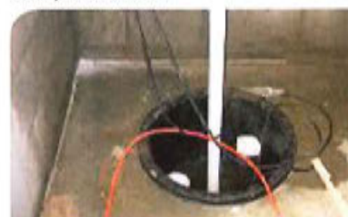
Photo Credit: Innovative Foundation Solutions, LLC. completefoundationrepairsolutions.com
