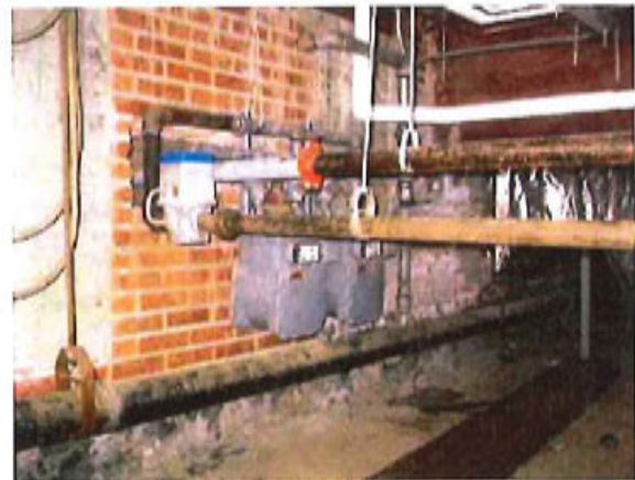
Figure 6. Crawl Space beneath 1st Floor
