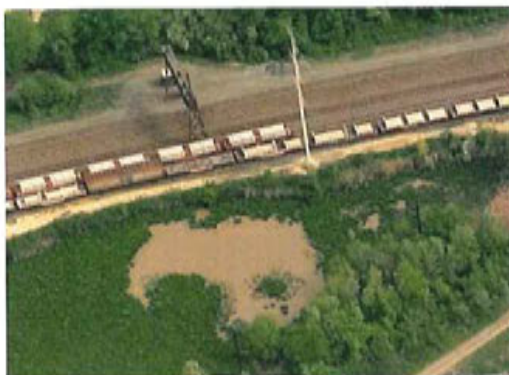
Figure 42. Lowlands with Water Adjacent to Tracks (MP 24.0 to 24.5)
