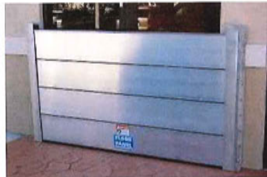
Figure 28. Emergency Flood Door Covering (Flood Panel, n.d.)
