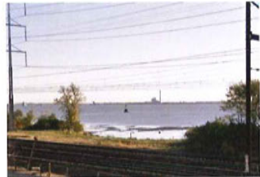
Figure 40. Low Elevation Tracks Adjacent to Delaware River (MP 21.0 to 21.5)
