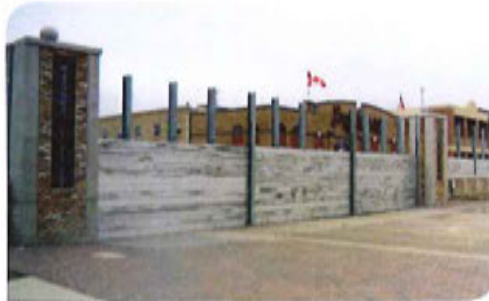
Photo Credit: Flood Control America, LLC floodcontrolam.com/projects/flood-wall-east-grand-forks
