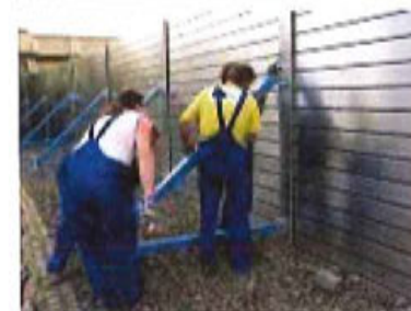
Figure 10. Installation of a Deployable Wall
