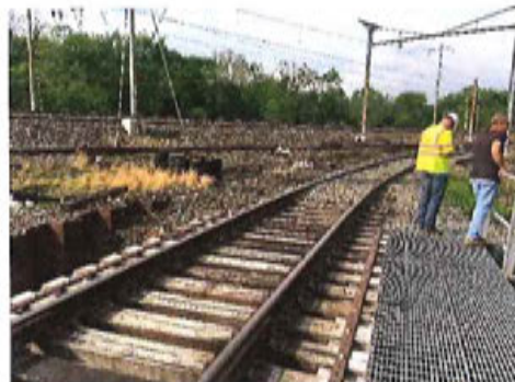
Figure 5. Track Section at the Wilmington Shops
