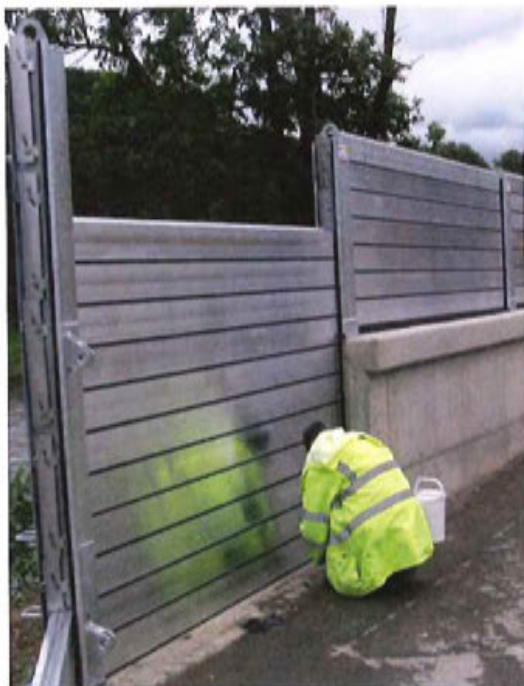
Figure 31. Semi-permanent flood barrier installation
